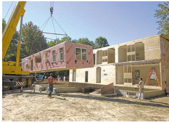
Modular construction often shortens the timeline and lowers the cost of the process.
